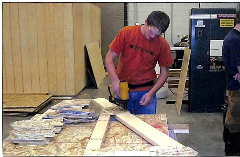
GUNNER: Roman Wolfley fires nails into a rafter in an effort to reinforce the gusset over the joint.
