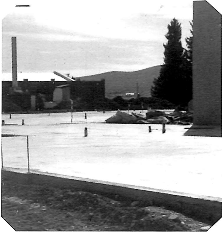
The foundation is laid!
