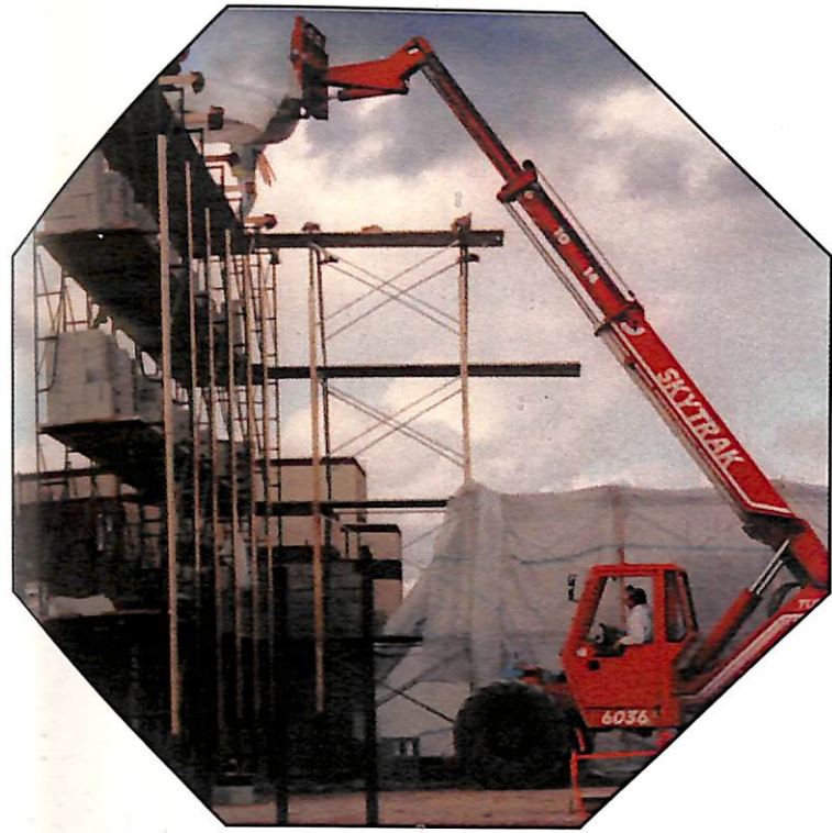
The crane helps to build another part for our new school!
