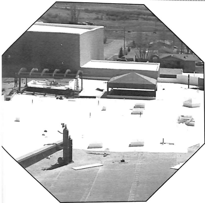
The roof is ready.
