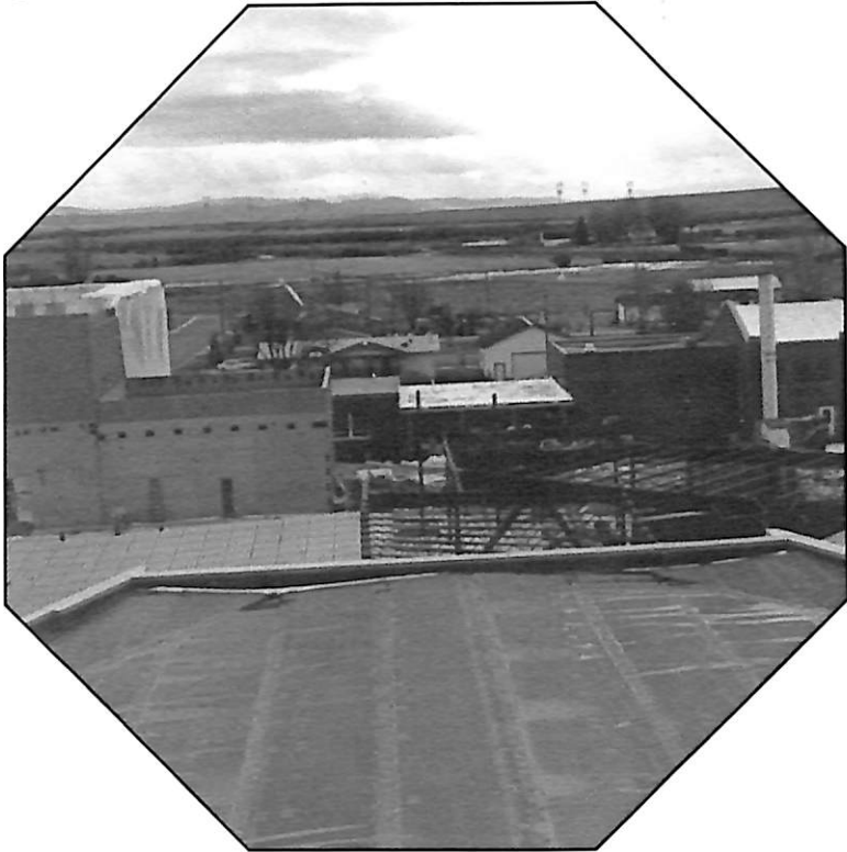
Laying The Roof.
