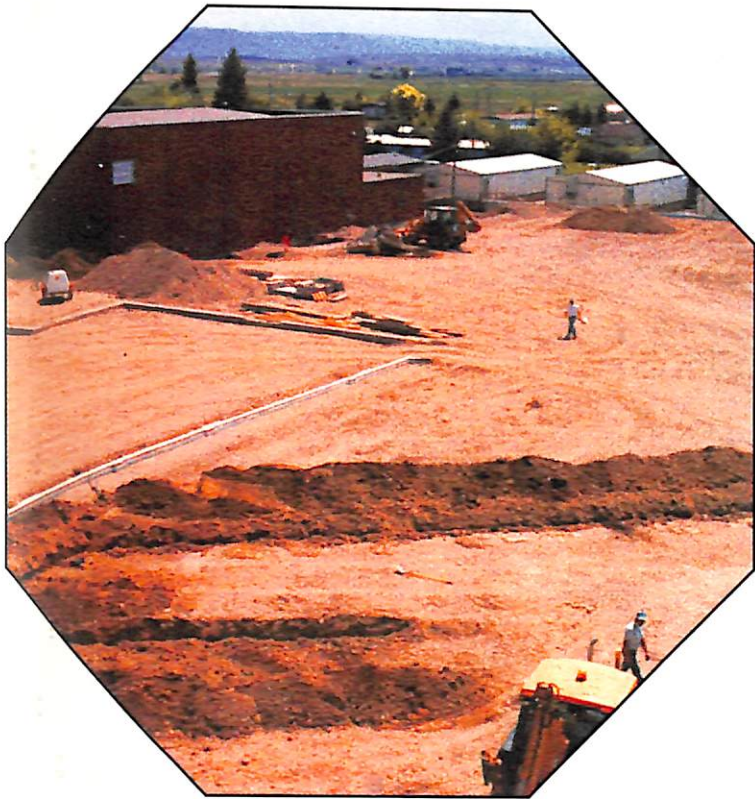
Ground breaking for our new school has begun!
