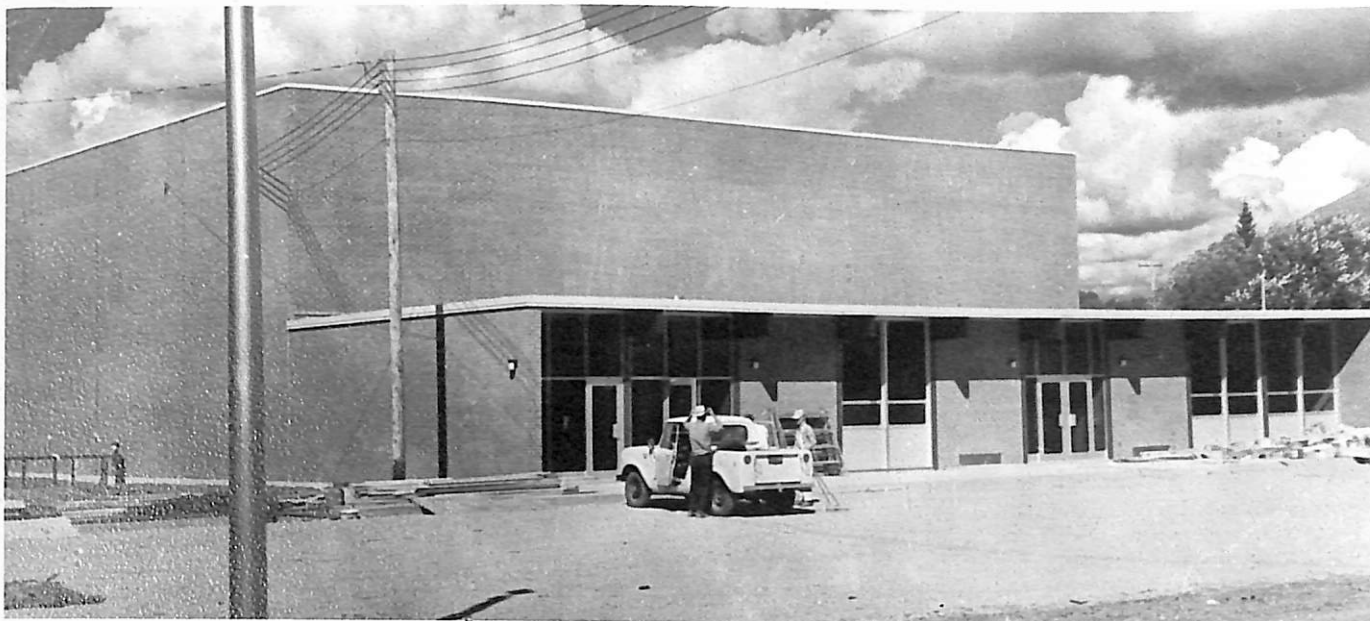
Southern view of new gym right after completion.
